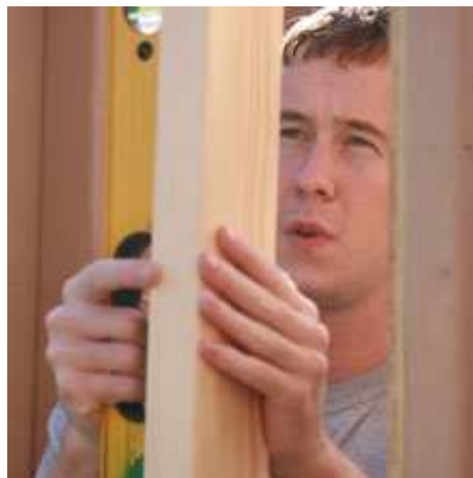
After gutting flooded homes in Cedar Rapids, Kerr helps reframe damaged walls.
